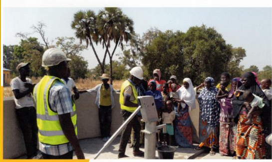
2022: Pumpbrunnen in Awonda (Togo)
